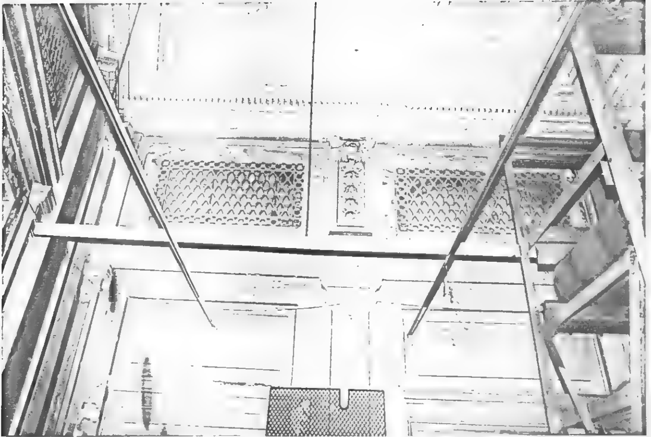
Ventilation grids appear on western wall of ferry concourse, dividing it from the railroad offices to the west.
